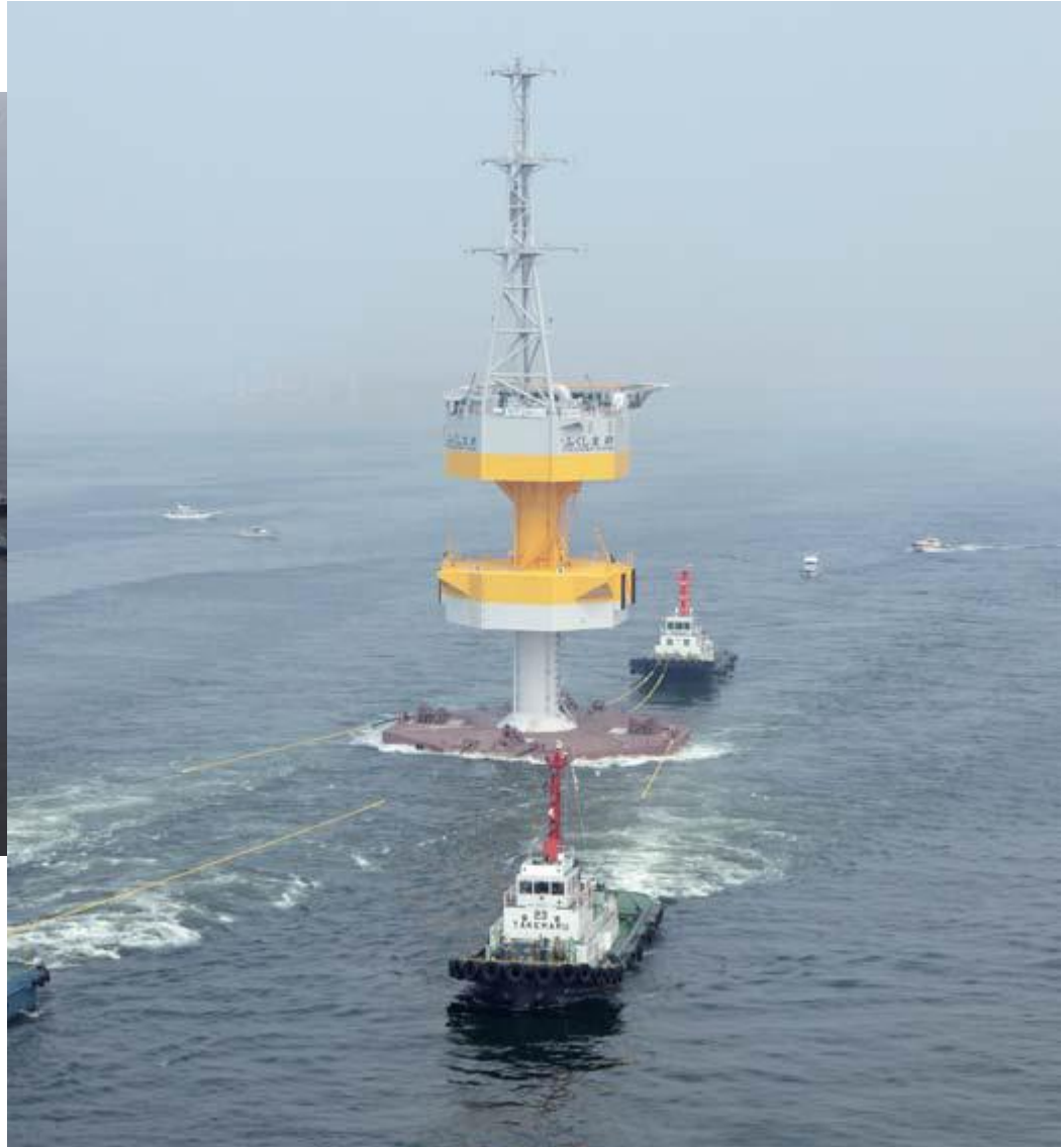
Transportation of floating sub-station
