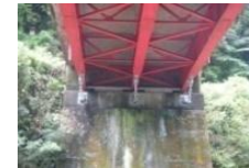
橋梁の耐震補強
