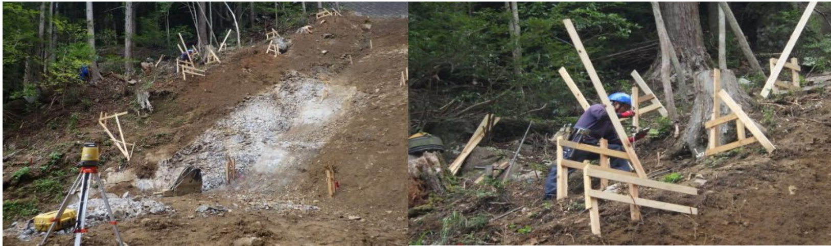
治山工事丁張設置
