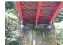
橋梁の耐震補強
