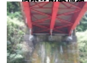
橋梁の耐震補強
