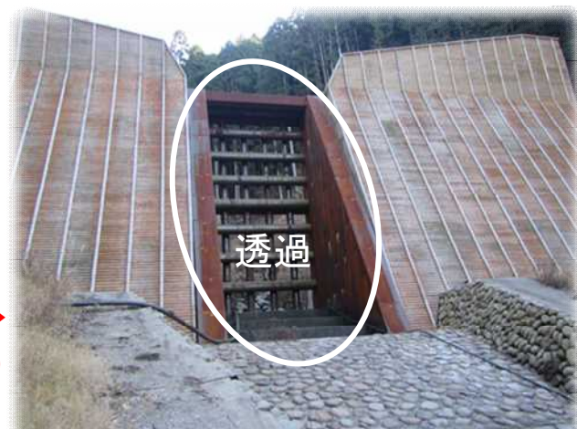
透過型砂防堰堤→ (安芸郡馬路村樋ノ口谷川)
