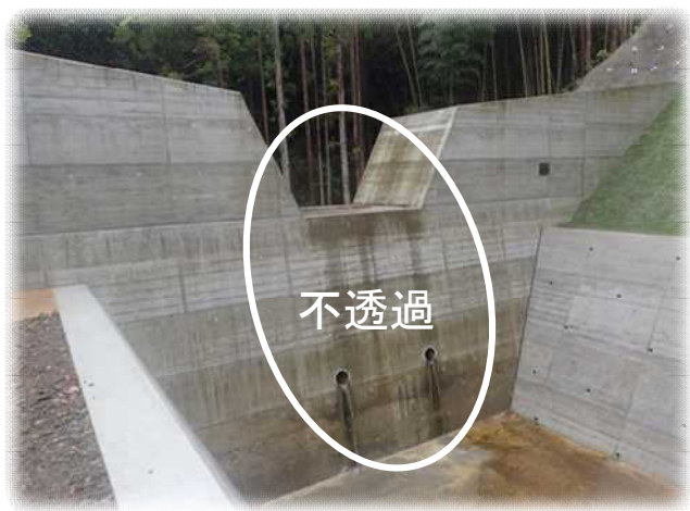
←不透過型砂防堰堤 (幡多郡黒潮町伊与喜谷川)
