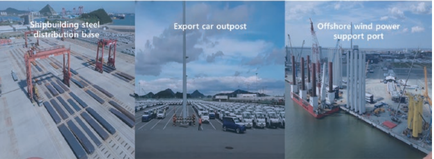
The Southwest Logistics Center Contributing to Regional Economic Development "Mokpo New Port"
